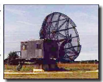
supposition that those structures were gigantic search lights. In fact, they were steerable UHF antennas, subsequently identified as such in aerial photographs taken in RAF reconnaissance flights by skilled Spitfire pilots diving at 300 mph through intense low level antiaircraft fire to an altitude of only fifty feet for oblique photography.
